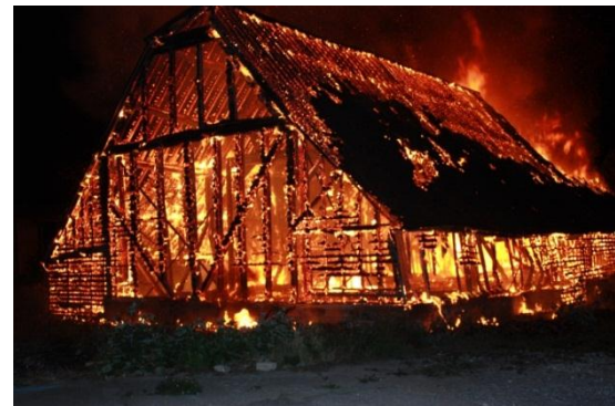
Figure 28: A timber frame building quickly destroyed by fire
