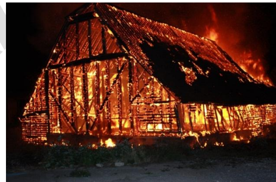
Figure 25: A timber frame building quickly destroyed by fire
