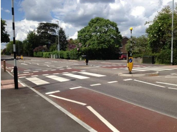
3.5.8 A new type of crossing for cycle users is now available. A Parallel crossing provides a crossing for cycle users alongside a traditional zebra crossing, and is sometimes referred to as a Tiger crossing
