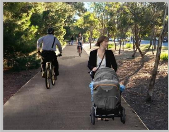
3.4.9 Usage should dictate the width of such paths, with 3 metres the recommended width, 2.5 metres the minimum. Paths wider than 3 metres should normally be segregated rather than shared.
