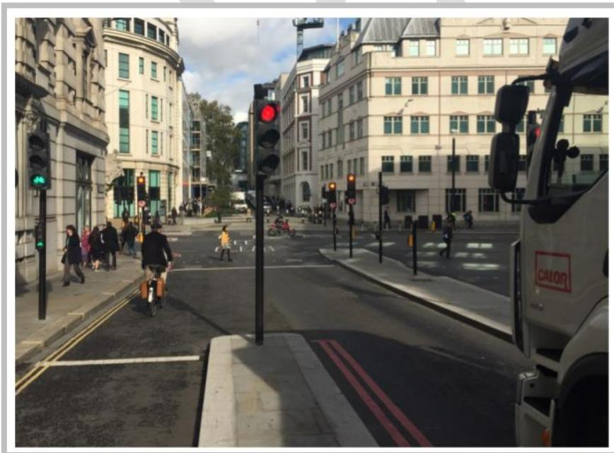
3.3.3 The toolkit for junction designers has recently been enhanced with low level signals for cycle users, early release for cycle users and two stage turns now
